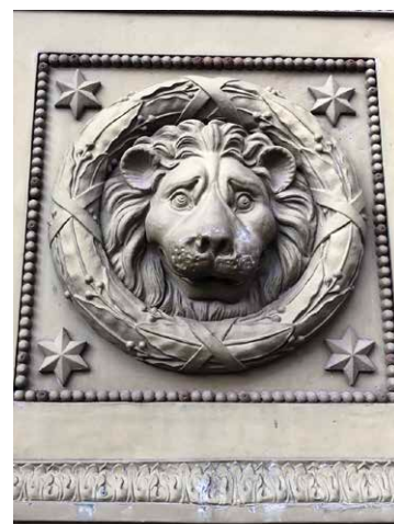
56. Doors of the General Staff Building in St. Petersburg, arch. Carlo Rossi, 1830. Photo: Vladimir Levin, 2019.
